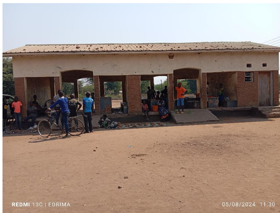
Figure 1: Market Shelter in GVH Mbenje (Source: Department of Physical Planning, 2024)
